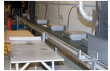
Once material is chopped to varying sizes as dictated by the computer's cut list, sort stations push the lengths automatically to sort tables.
